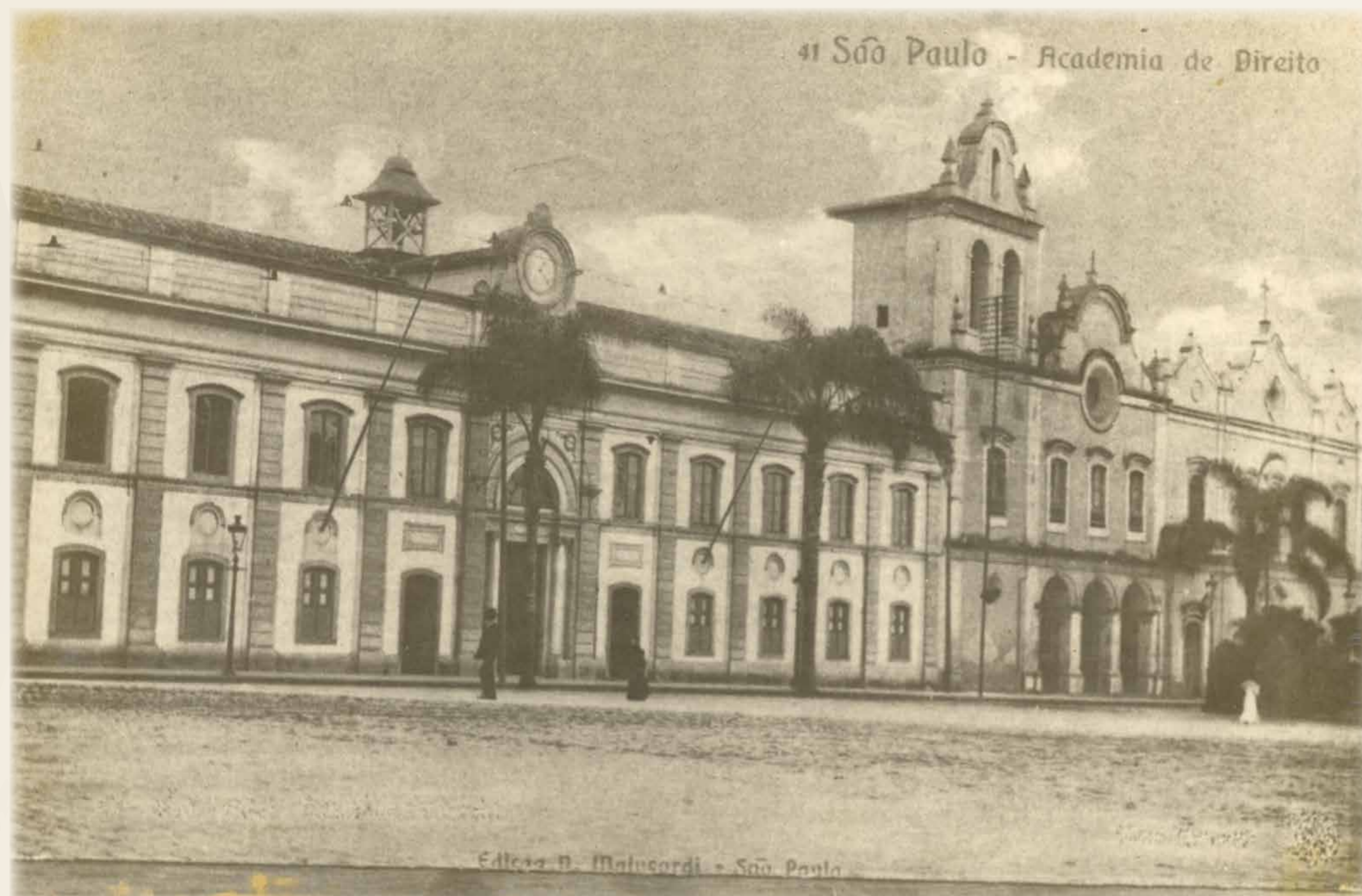
Building where the São Paulo Law School was located and which had previously been the convent of the Seraphic Order of St. Francis of Assis.
